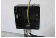
**18.** Make connections as shown in the following figures. Connect the power wires with the cable wires. Connect the incoming ground wire with the cable braid. The wire nuts, included, must not be connected with aluminum wires. The junction box also needs to be grounded.
