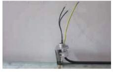
**17.** Use a metallic junction box to ensure a proper grounding. Insert and tighten the heating cable. **NOTE:** Leave at least 6" of lead wire inside a junction box.
