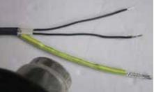
**12.** Slide "black shrinkable tube" of 1"(25mm) on the end of heating cable.
