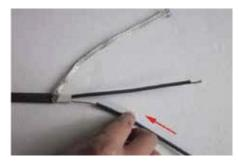
**10.** Carefully shrink the tubes by heating from side to side continuously, being careful not to damage heating cable.
