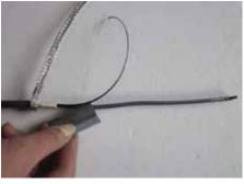
7. Peel back exposed wires from PTC material.
